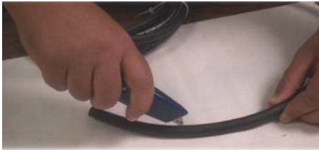
Figure 4.15 Strip the outer jacket
